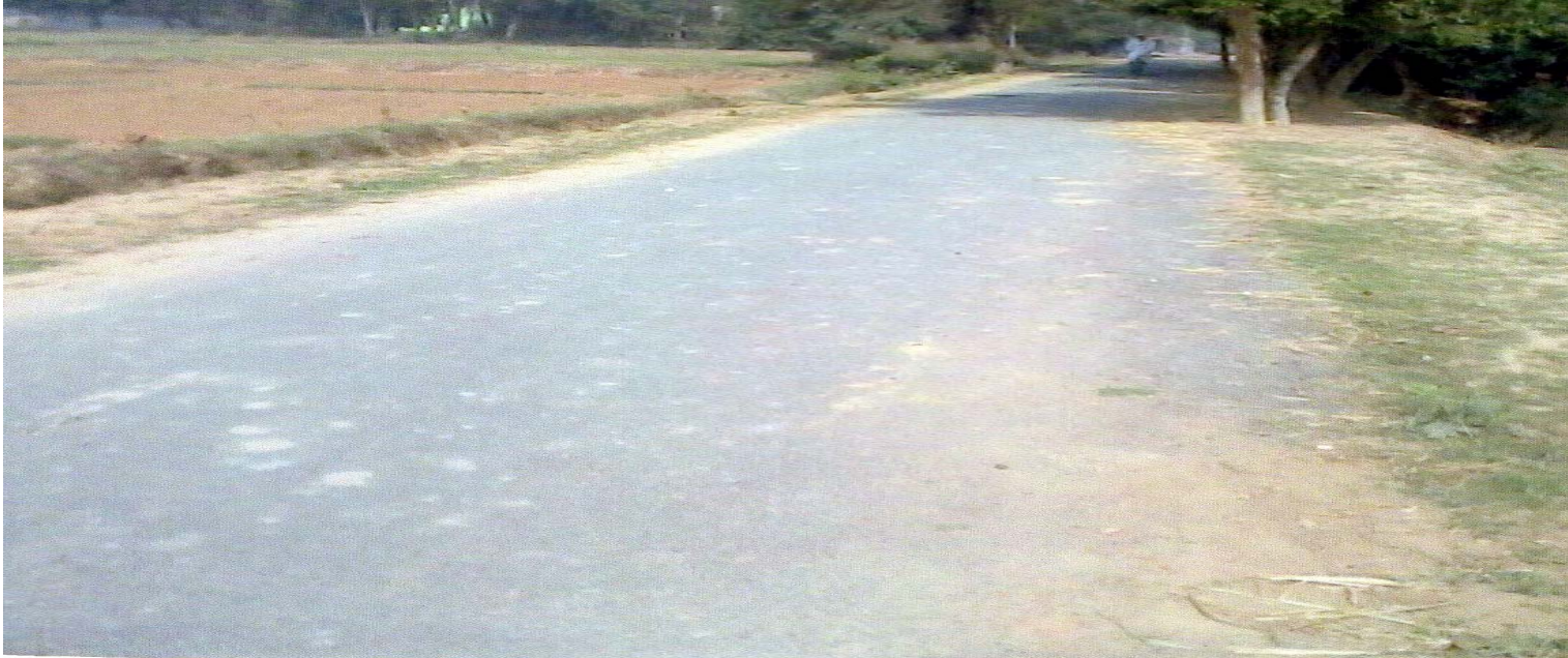
PWD – Village Barthapur, habitation- Pandit purwa
